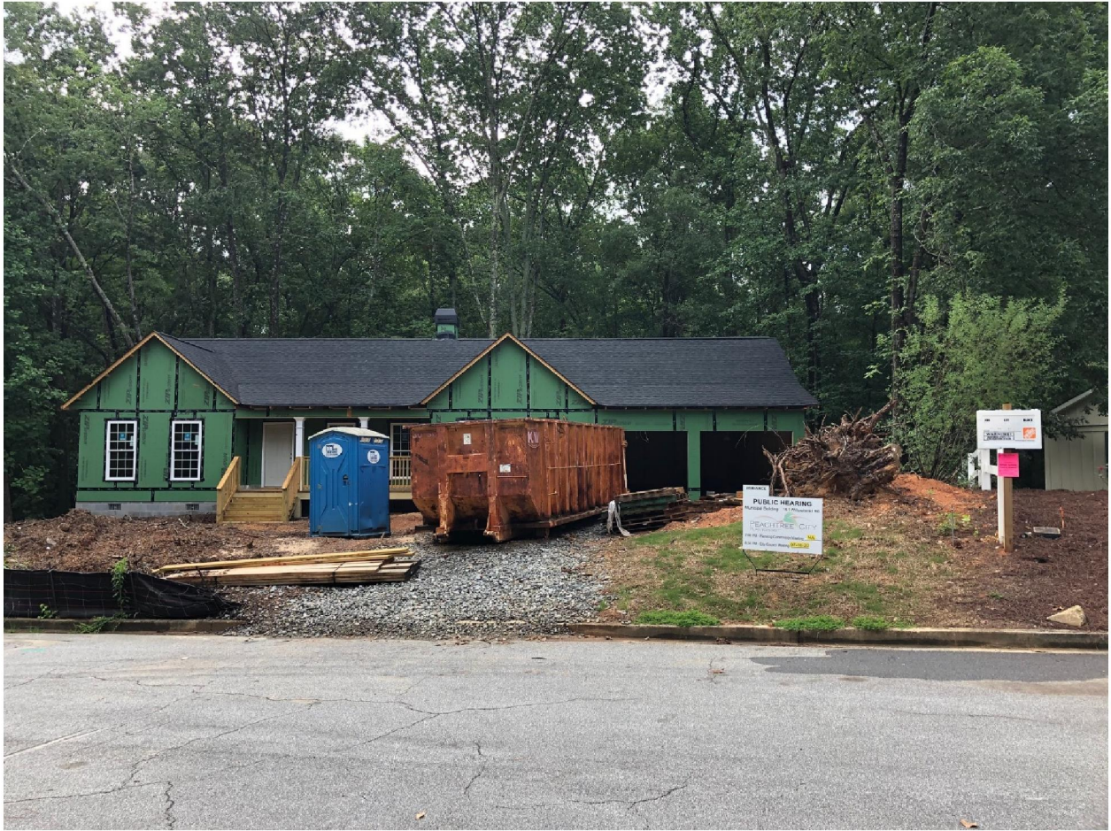
Figure 1: House under construction at 102 Arrowhead Ct
