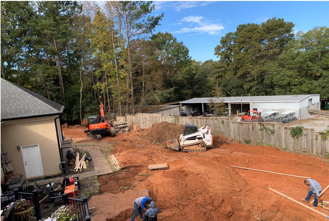
Figure 2: View from rear deck of 104 Country Club Court
