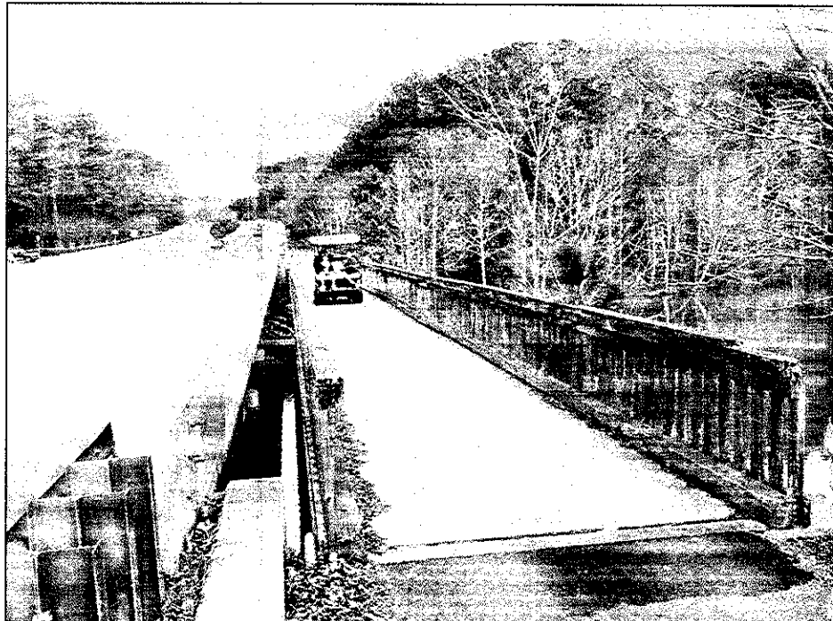
Figure 1. – Golf Cart Crossing Bridge
