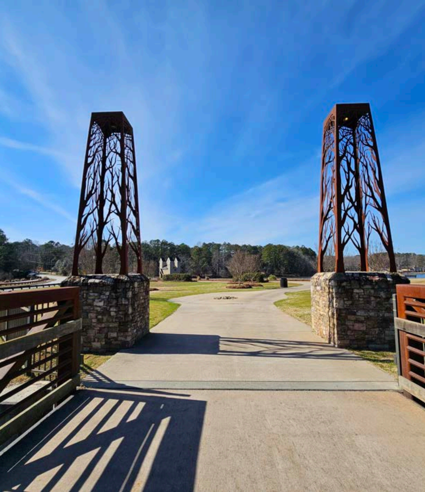
Lake Peachtree Dam & Spillway Park
