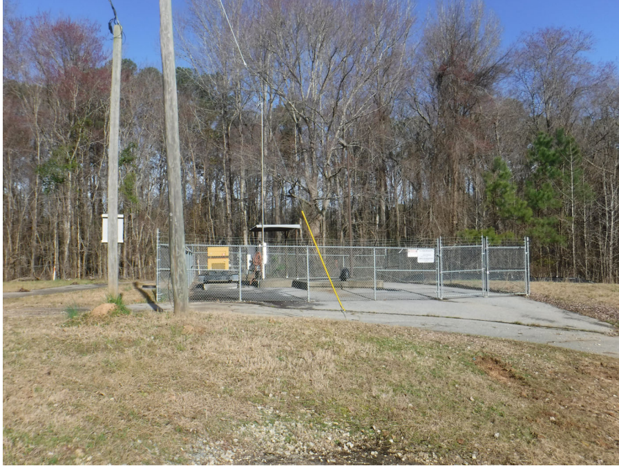
Subject Lift Station
