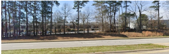
View of East Facade from HWY 74 - Winter
