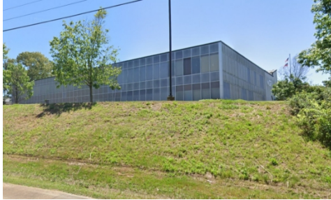
Corner Facing HWY 74 - Existing
