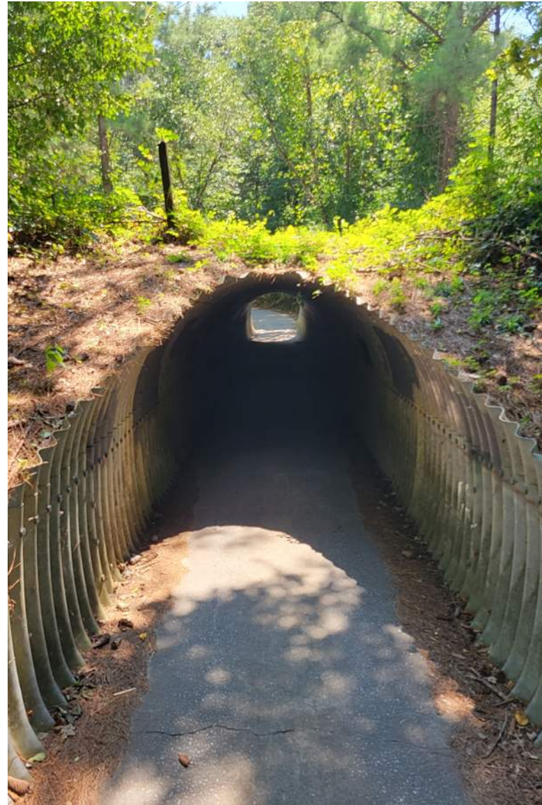
Tunnel 8 Western Approach
