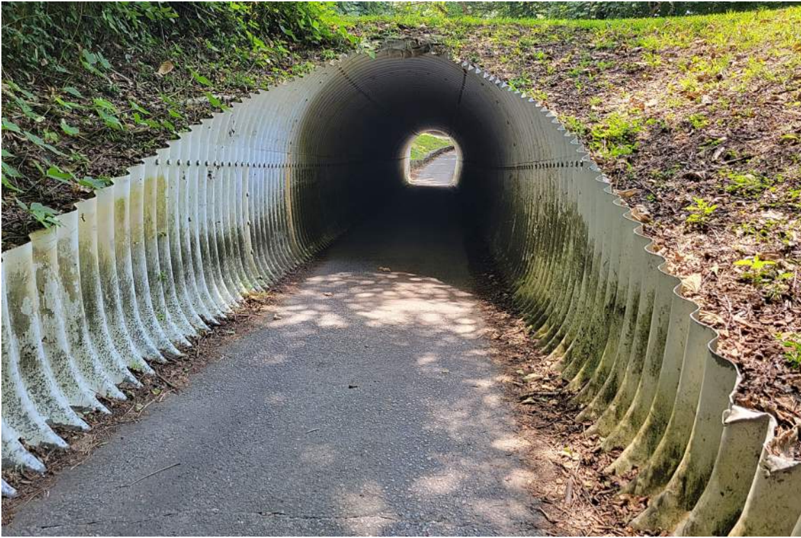
Tunnel 9 View from Northern Approach
