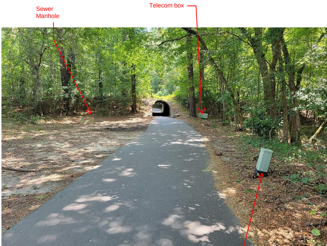
Tunnel 8 Eastern Approach
