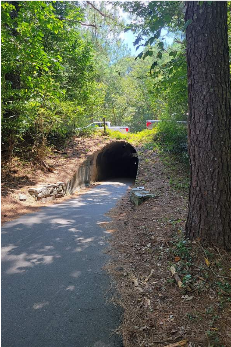
Tunnel 8 Eastern Approach
