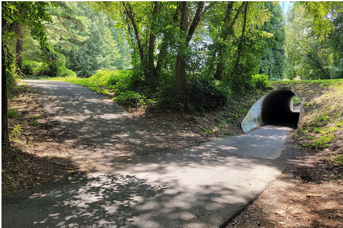
Tunnel 9 Northern Approach
