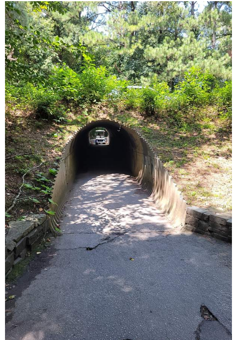
Tunnel 8 Western Approach
