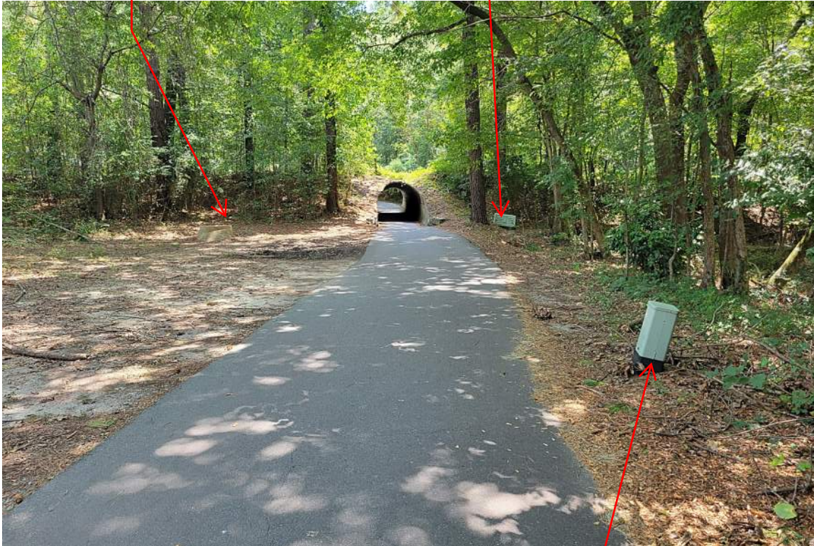
Tunnel 8 Eastern Approach
