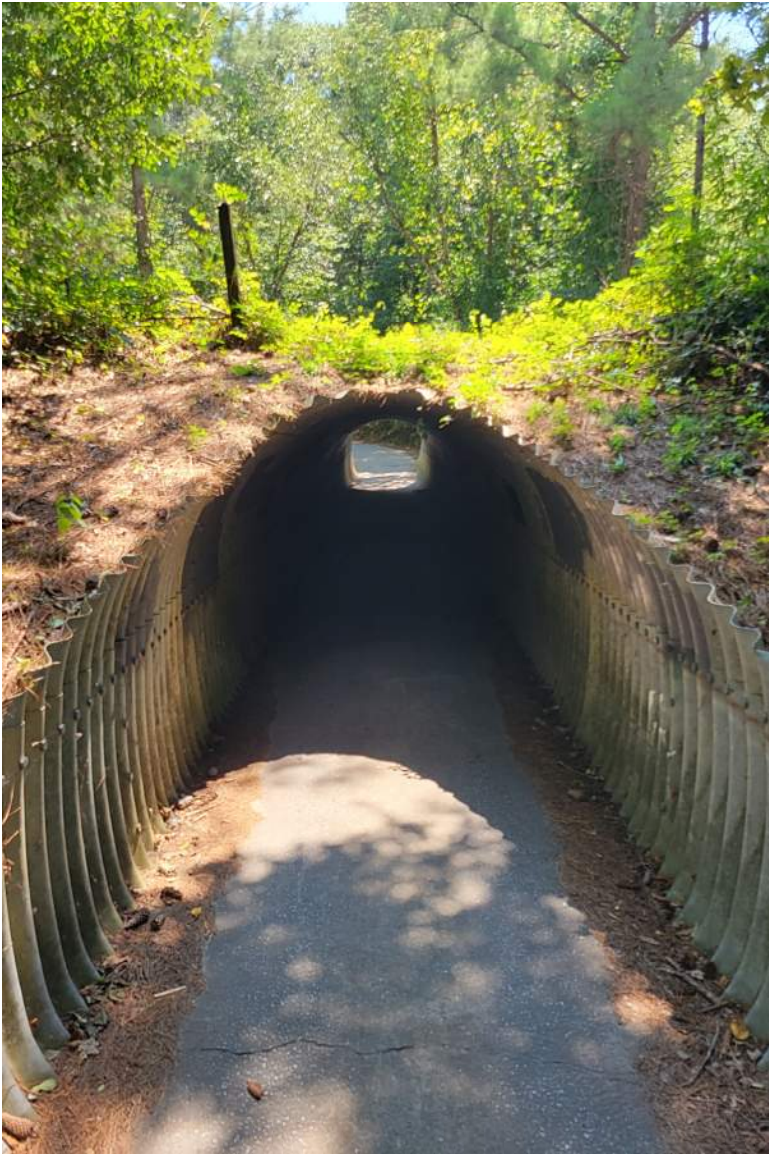
Tunnel 8 Western Approach
