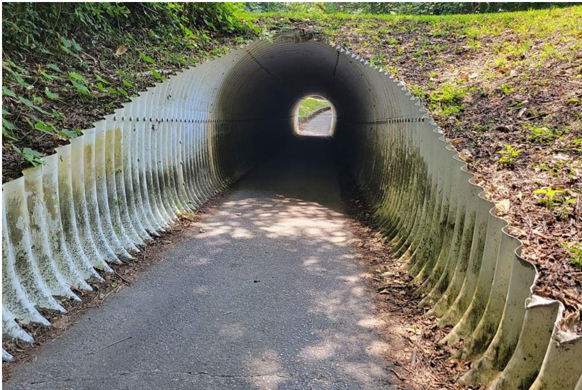
Tunnel 9 View from Northern Approach
