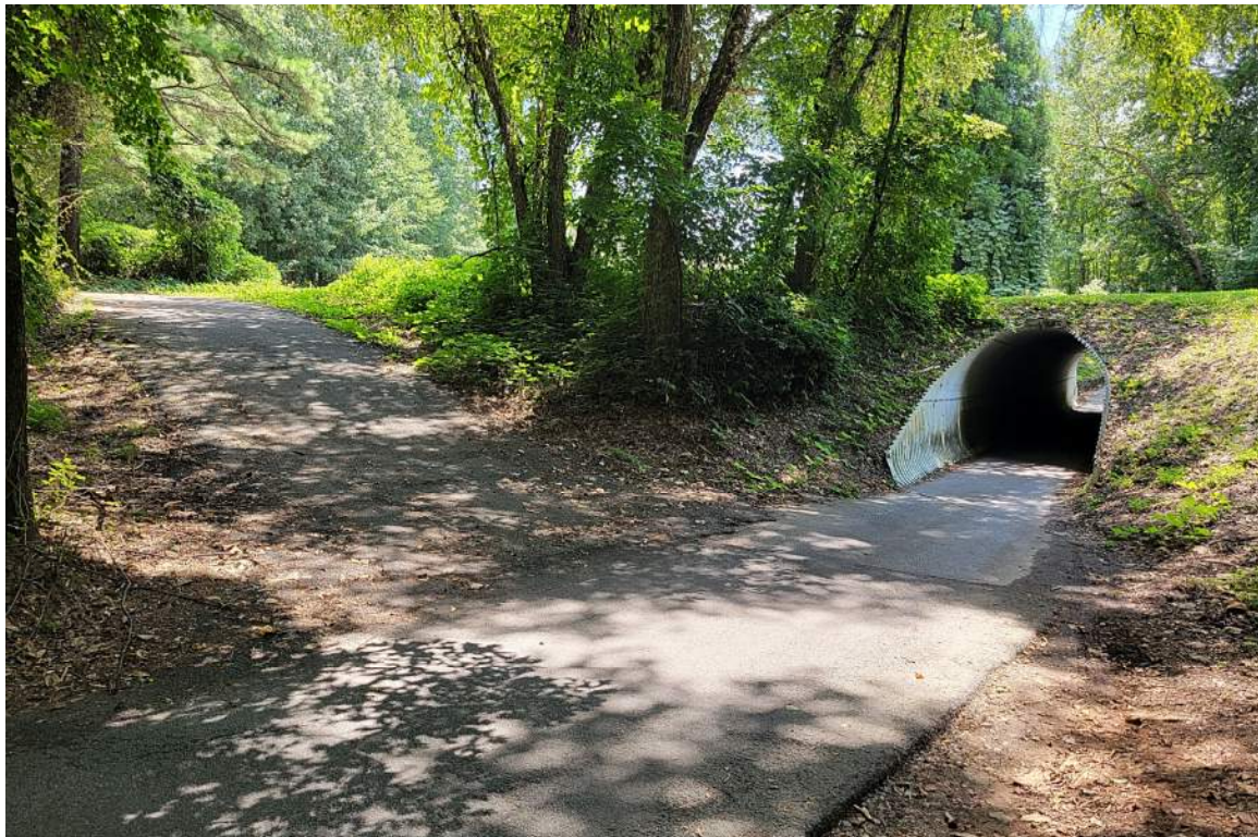
Tunnel 9 Northern Approach
