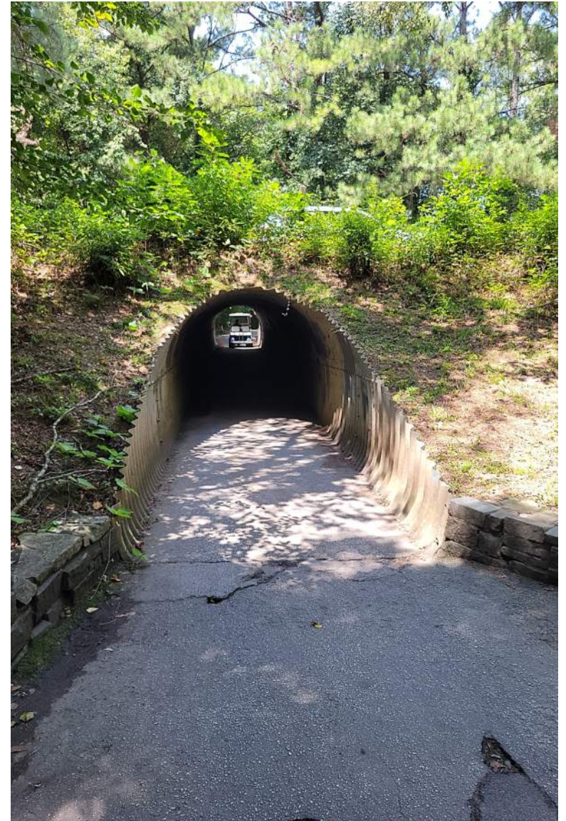
Tunnel 8 Western Approach
