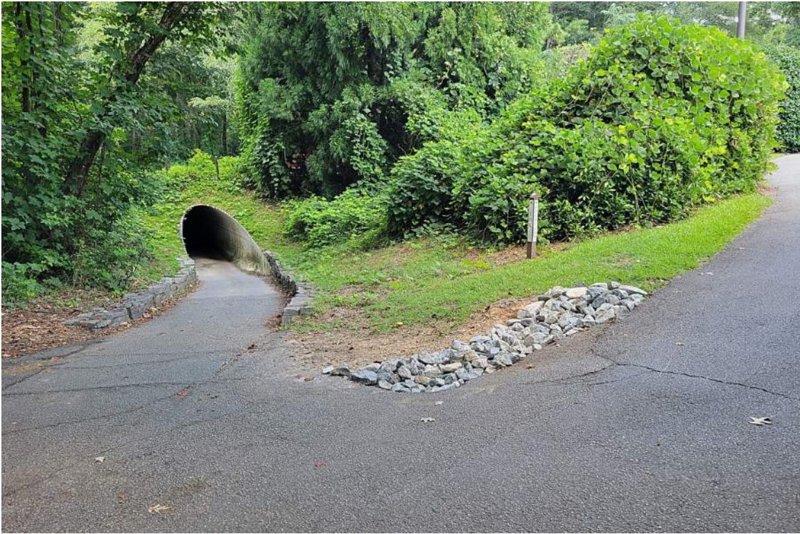
Tunnel 9 Southern Approach
