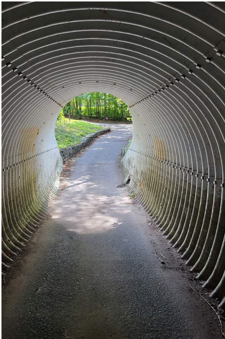
Tunnel 9 View from inside tunnel towards steep Southern
