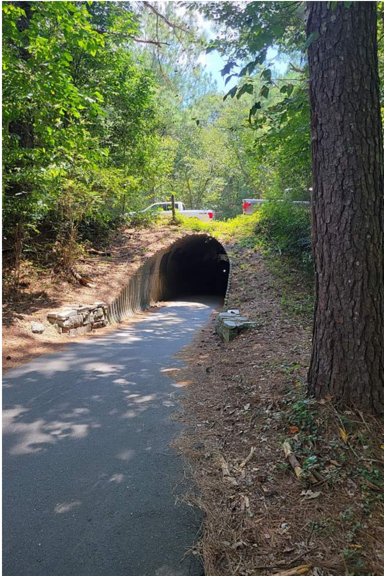
Tunnel 8 Eastern Approach
