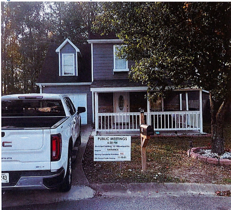
Figure Two: Picture of front porch addition
