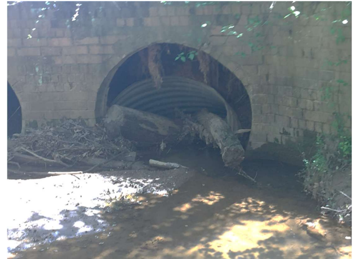
Road Sinkhole 5.5 FOOT diameter
