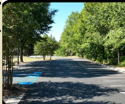
2025 PAC PAVING PROJECT
