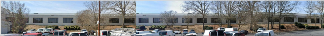
EXISTING STUCCO CORRIDOR ALONG HWY 74
