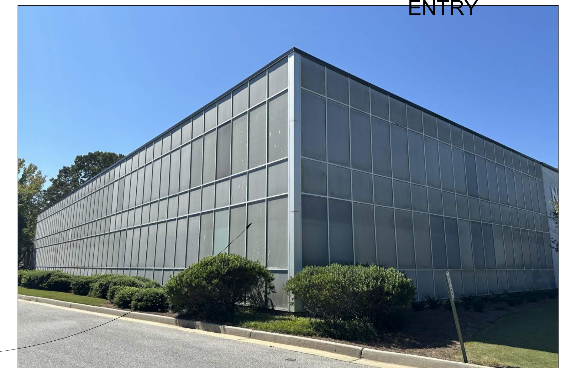
EXISTING CORNER FACING 74
