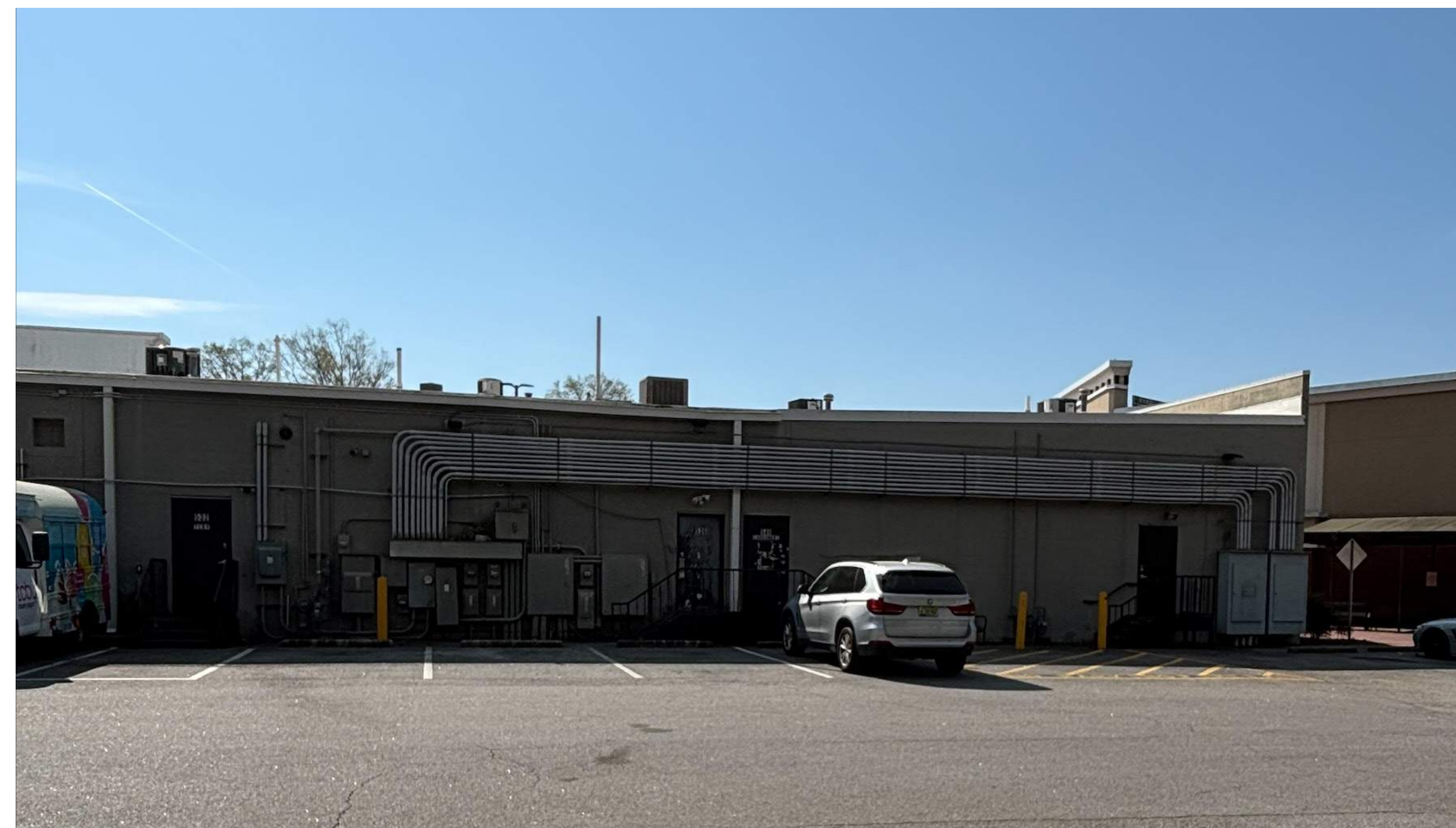
PHOTO 6 (USE AS REFERENCE FOR ENTIRE REAR)
