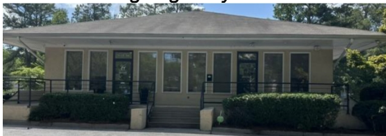
Facade facing Eastbrook Bnd
